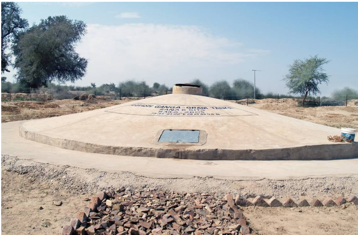
Photograph 3: Shared reservoir, 400,000 litres
